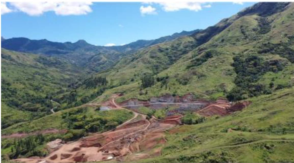
Photo 10: Tuvatu tailings storage facility looking north into Navilawa caldera
