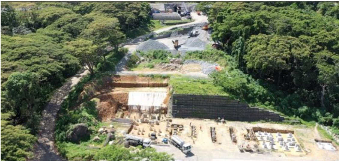
Photo 2: Aerial view of the Tuvatu production decline portal and plant site
