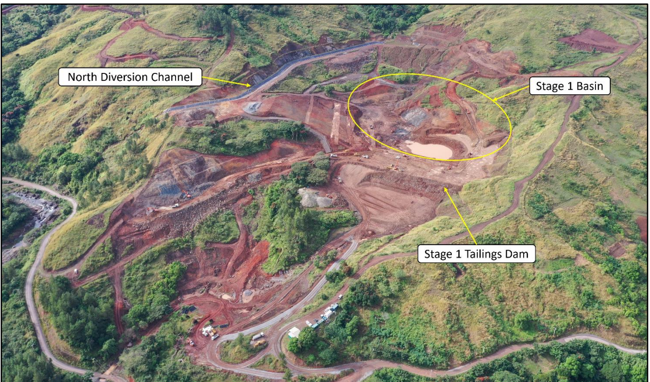
Figure 6. Aerial view of TSF under construction, June 16, 2023.
