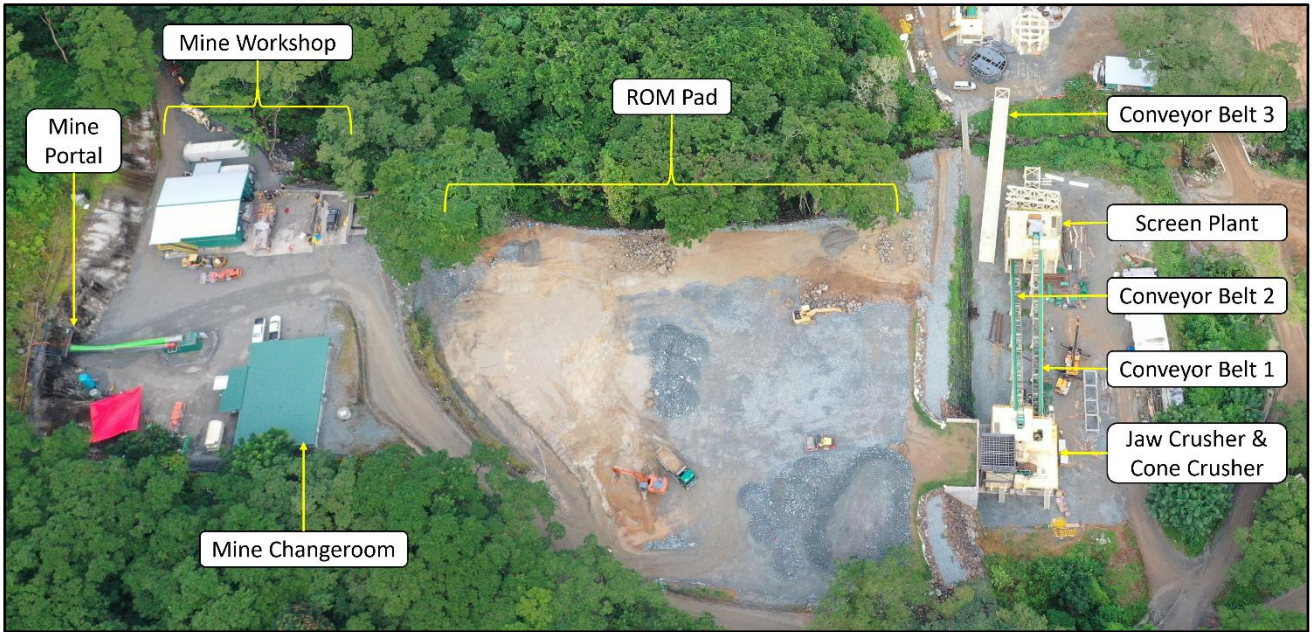
Figure 3. Aerial view of mine portal, ROM pad, and crushing plant, June 16, 2023.
