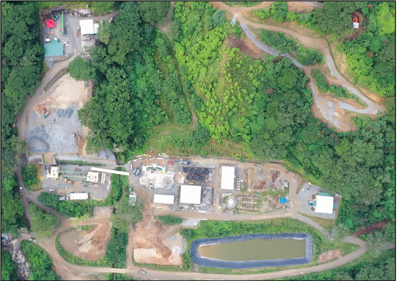
Figure 5. Vertical aerial view of mine site under construction, June 16, 2023.
