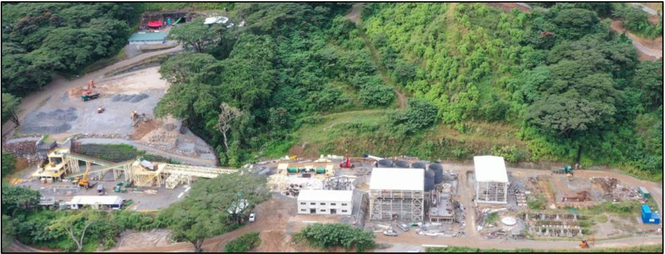
Figure 1. Tuvatu Gold Mine Under Construction. See below for additional images.
