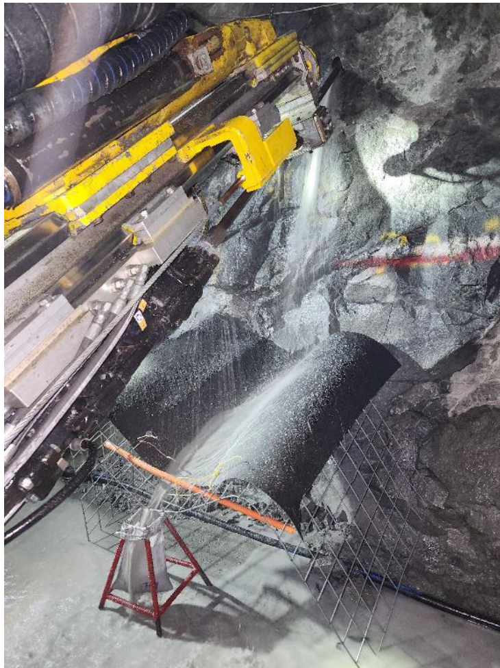
Figure 16.3 Tuvatu Underground Sludge Sample Drilling
