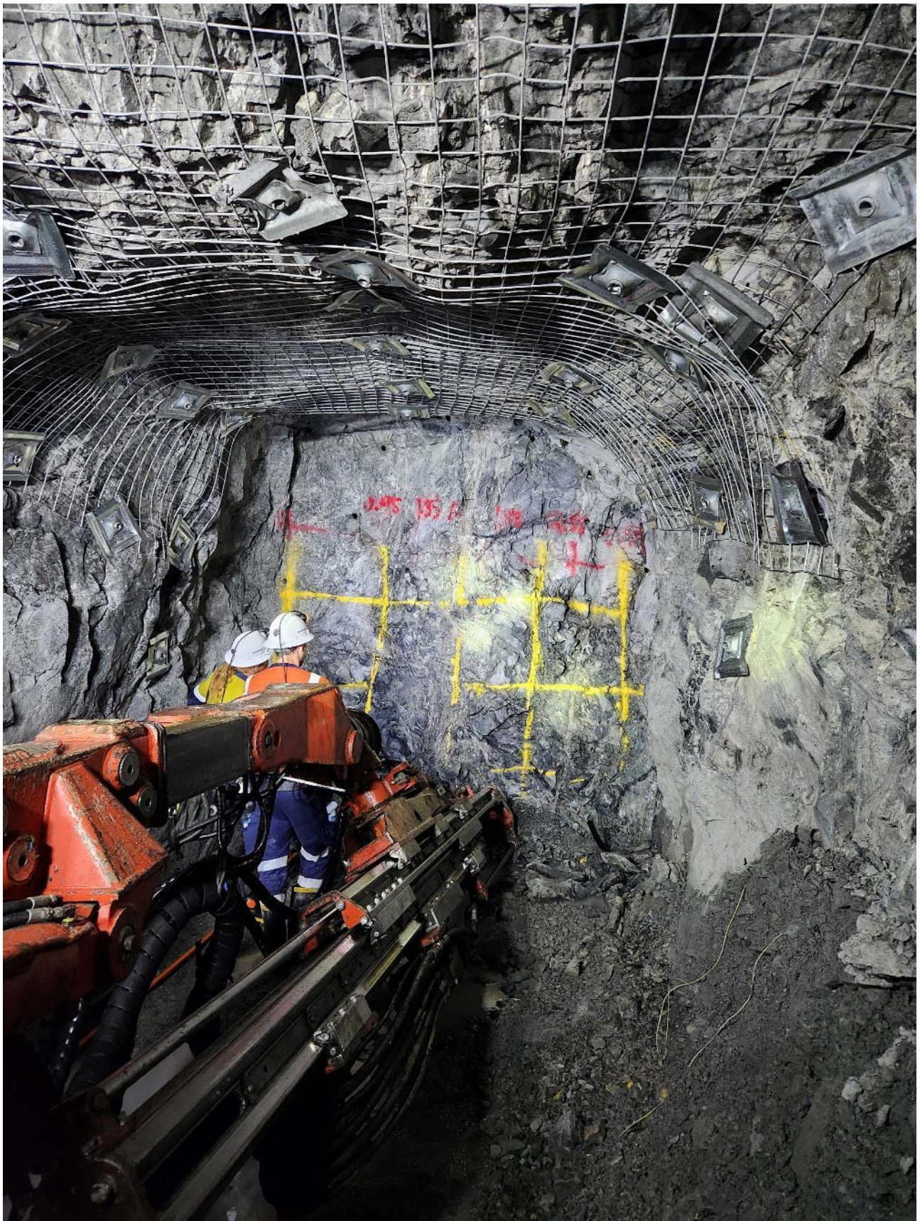
Figure 16.4 Tuvatu Underground Jumbo Development Drilling
